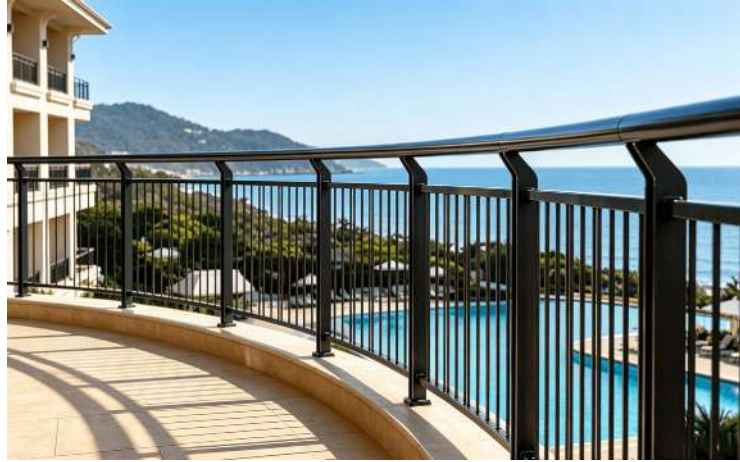
02 Metal Balcony Railing
