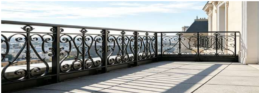
Galvanized Iron Balcony Railing
